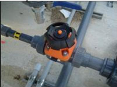
The RAD flow rate control valve is used to control bubble quantity and RAD flow rate into the DAF. The RAD by-pass valve is used to adjust pressure independently of the RAD flow rate. This way, RAD flow rate can be adjusted to achieve the bubble quantity desired and the by-pass valve is used to adjust pressure which affects bubble size. Generally speaking, lower pressure ~30 psu produces larger bubbles
